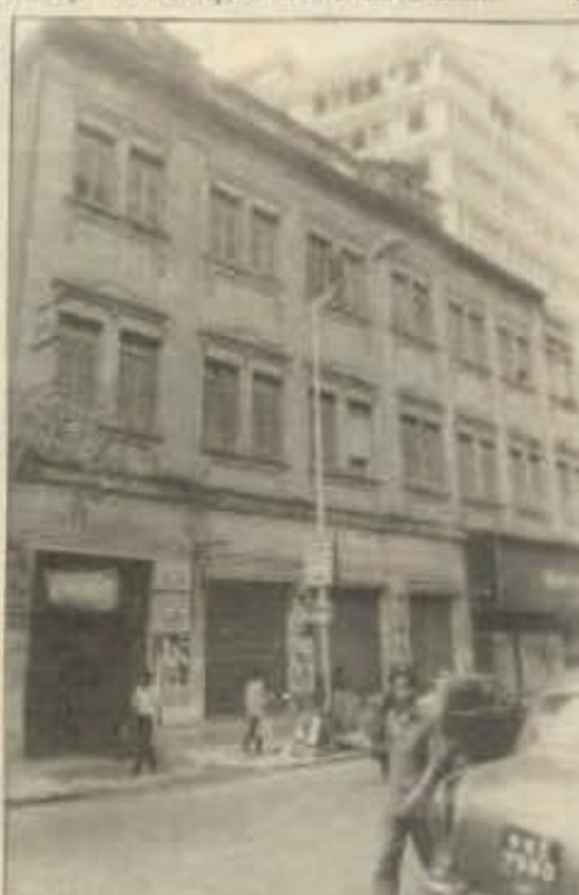
An old building on Park Street
